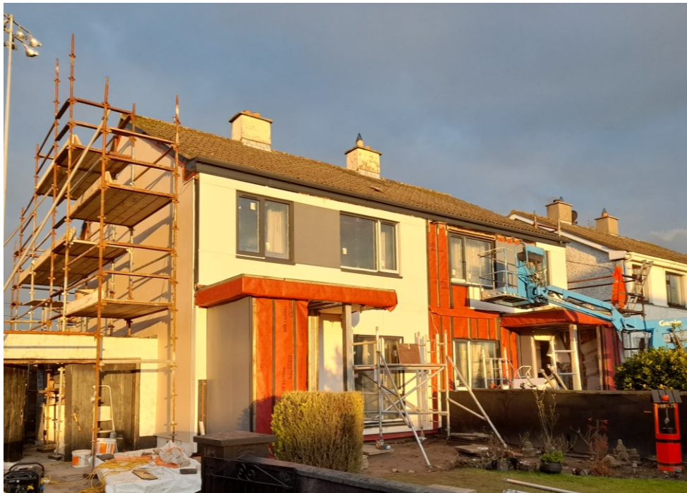
Retrofitting process for the Irish Demonstrator Case
